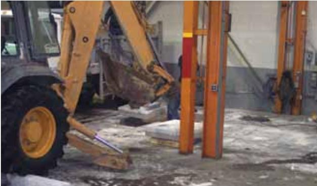
***The old foundation is being removed so a new and stronger foundation can be poured for two of the larger machines to be relocated.***
